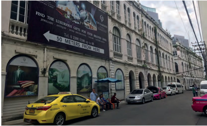
06 East Asiatic Company Building East Asiatic Company Building
